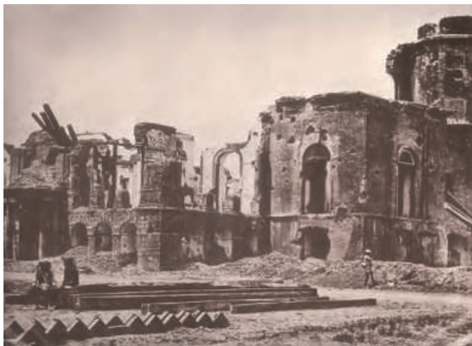
Fig. 17 – Ruins of the Residency in Lucknow
