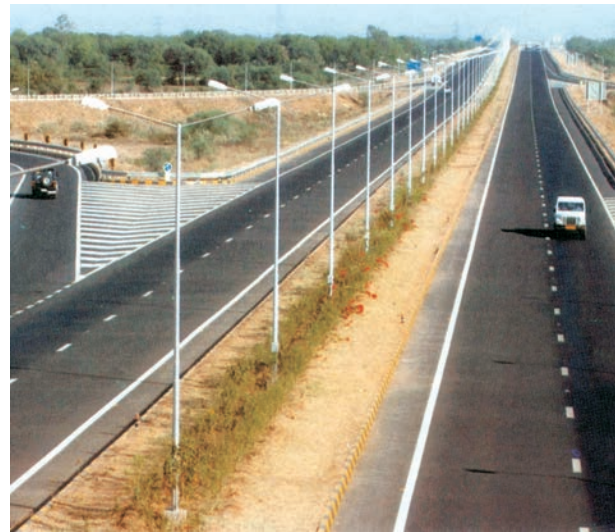
Fig. 7.2: Ahmedabad- Vadodara Expressway
