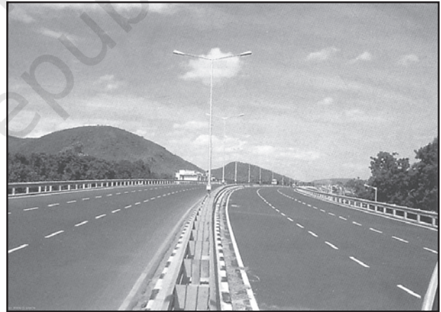
Fig. 7.3 : Dharmavaram Tuni National Highway, India
