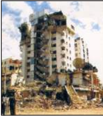
Fig. 3.3a: Destruction caused by an Earthquake in Gujarat
